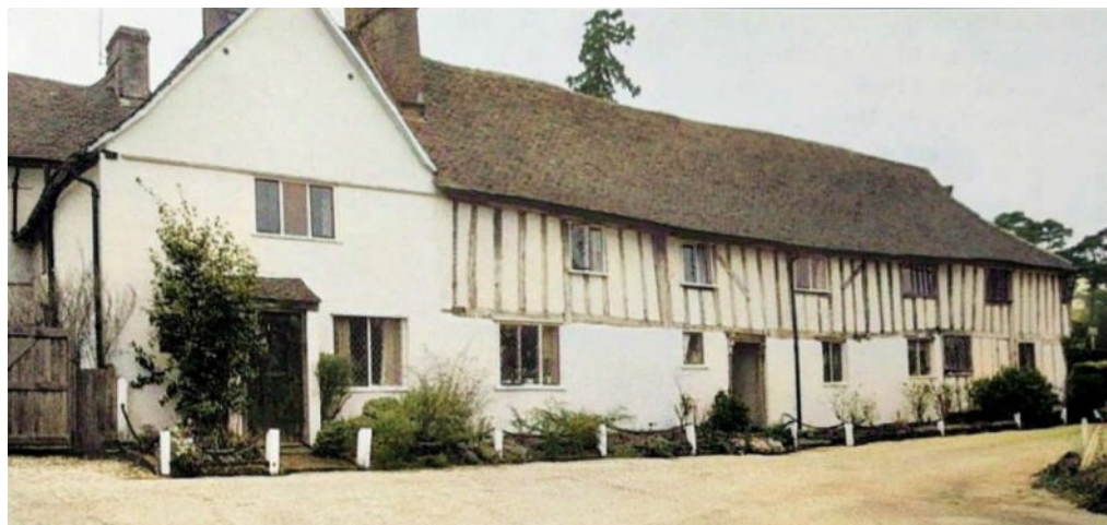
East Front after restoration.
