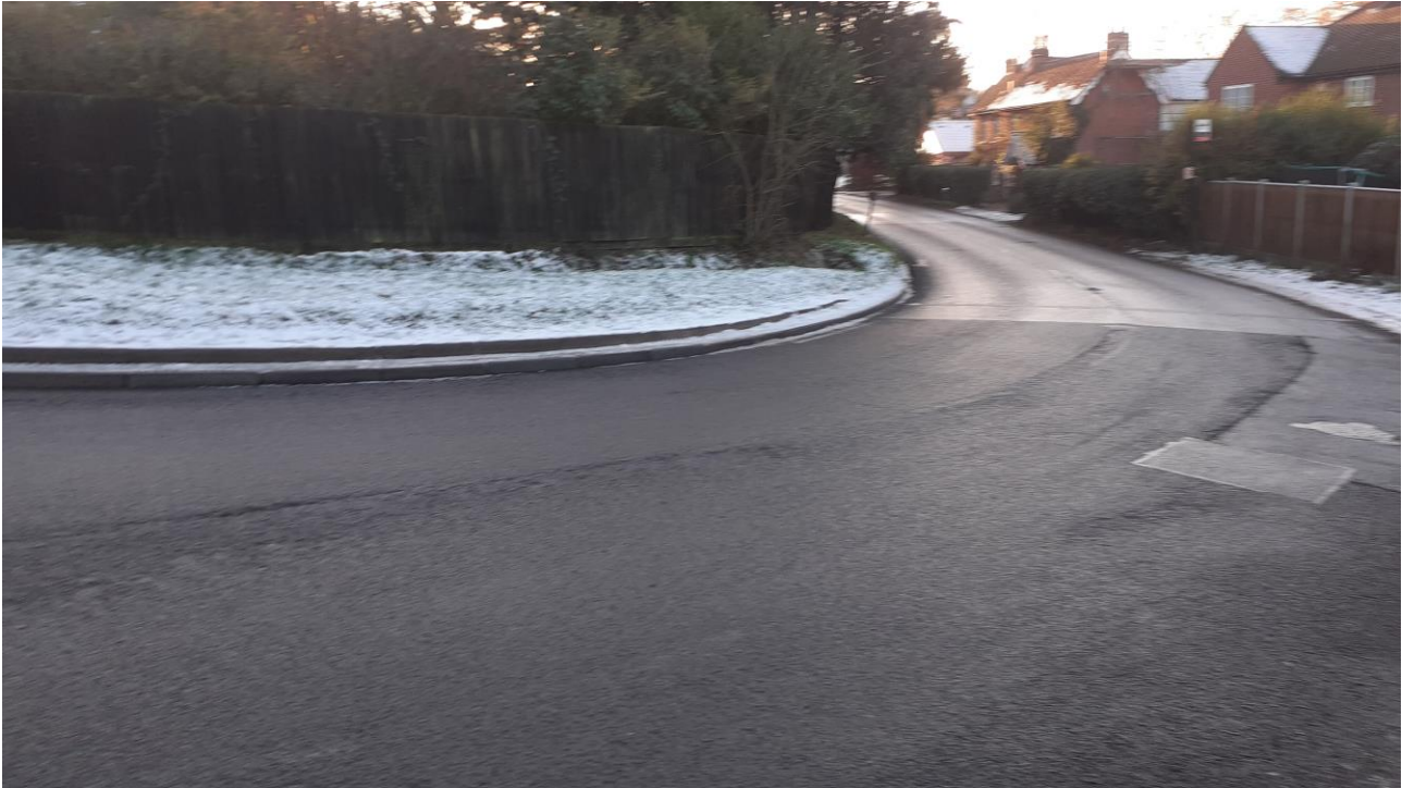
Figure 12: View back along Birchwood Road (ref: 20221215_145403). 54-03
