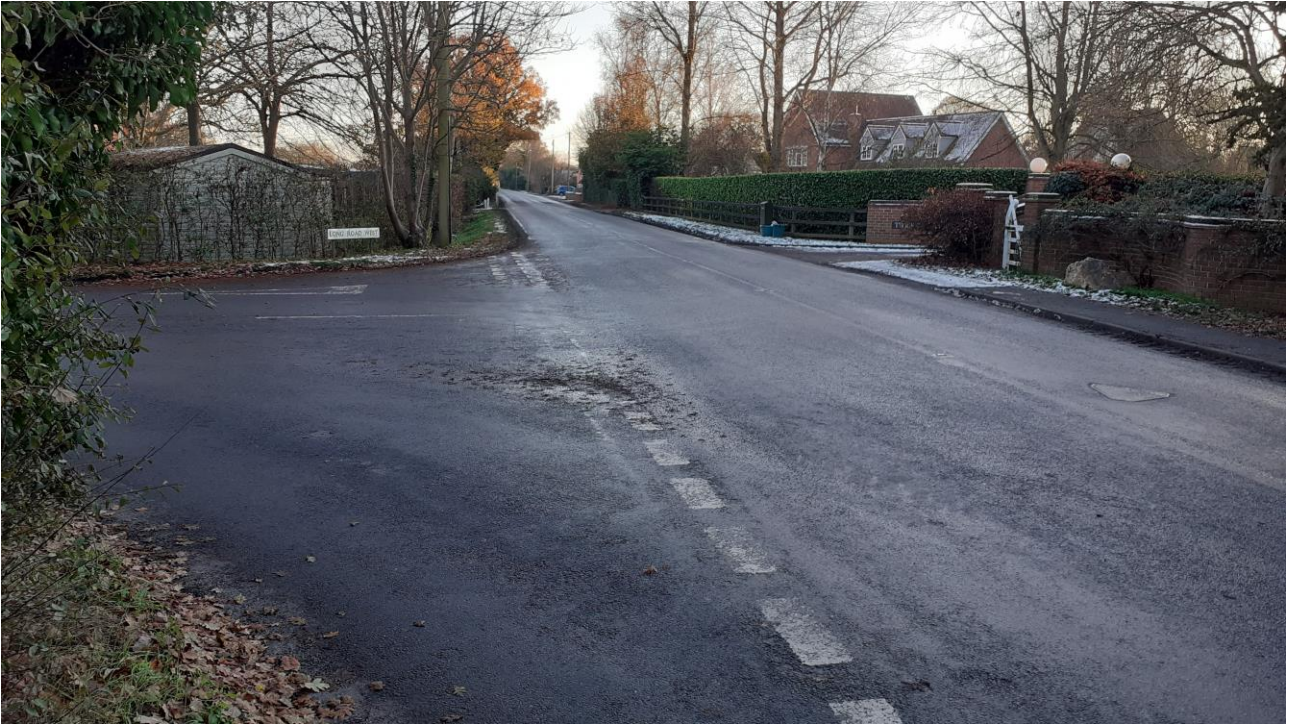
Figure 8: View of junction from Ardleigh Road (ref: 20221215_145755).
