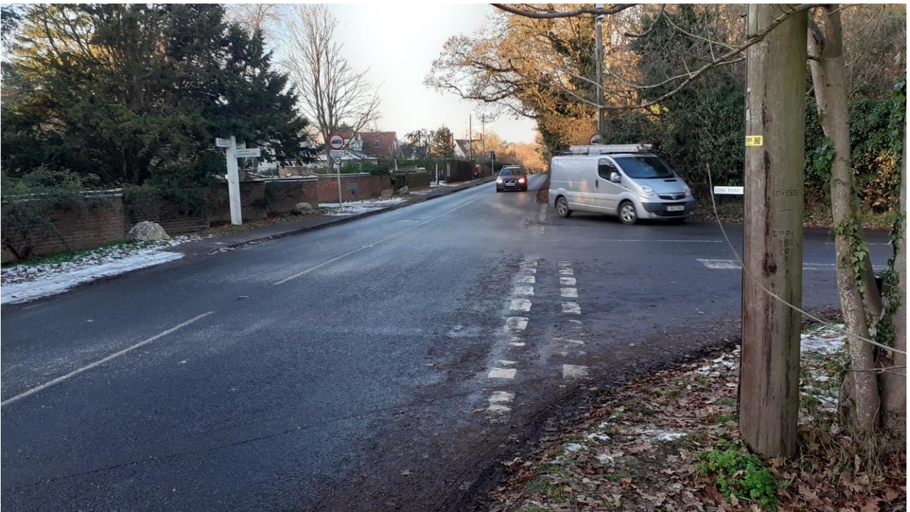
Figure 9: View of junction from Ardleigh Road (ref: 20221215_145651).
