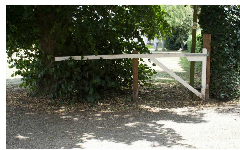
EXISTING BOOM SWING GATE AT CRICKET PAVILION CAR PARK
