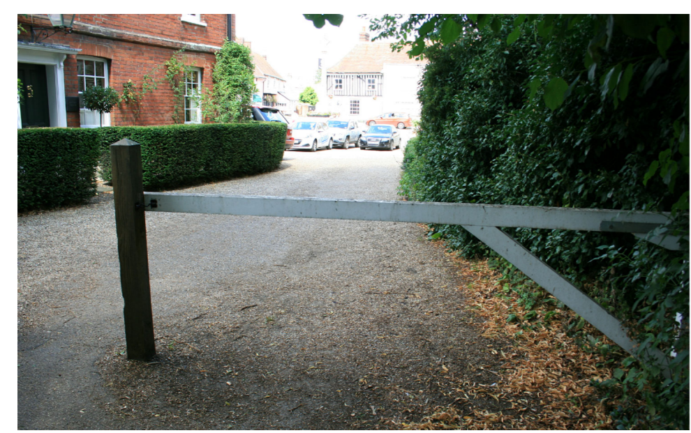
EXISTING BOOM SWING GATE AT ROYAL SQUARE
