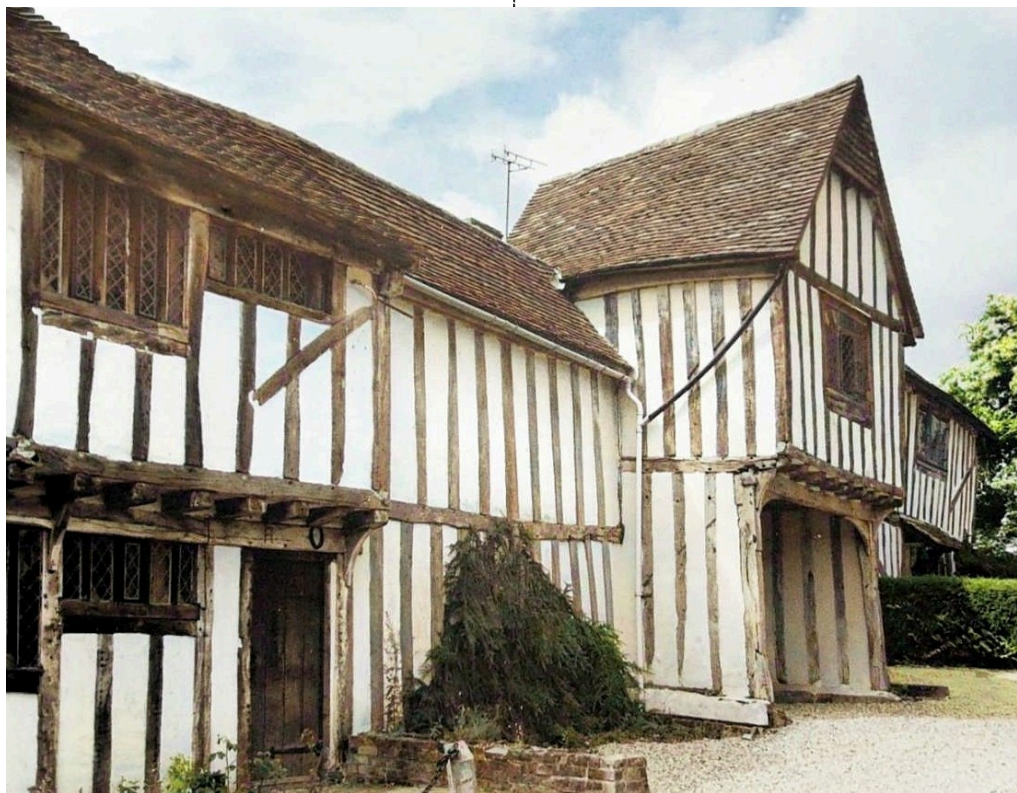
North side after restoration.
