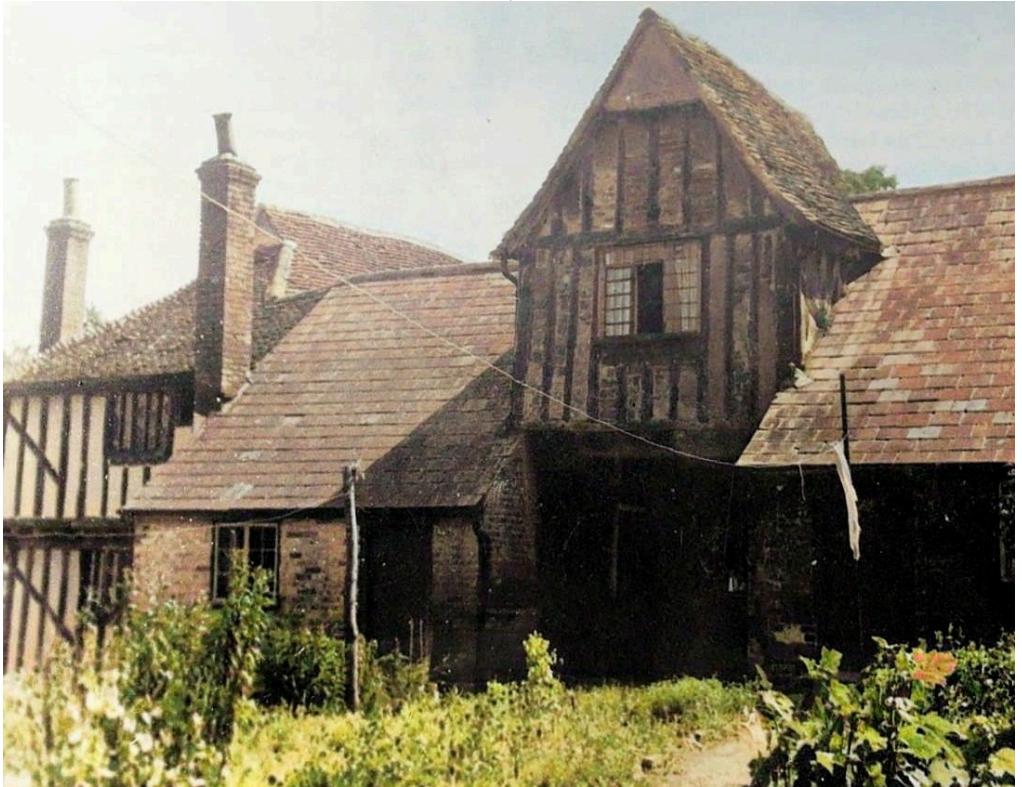
North side before restoration - 1952
