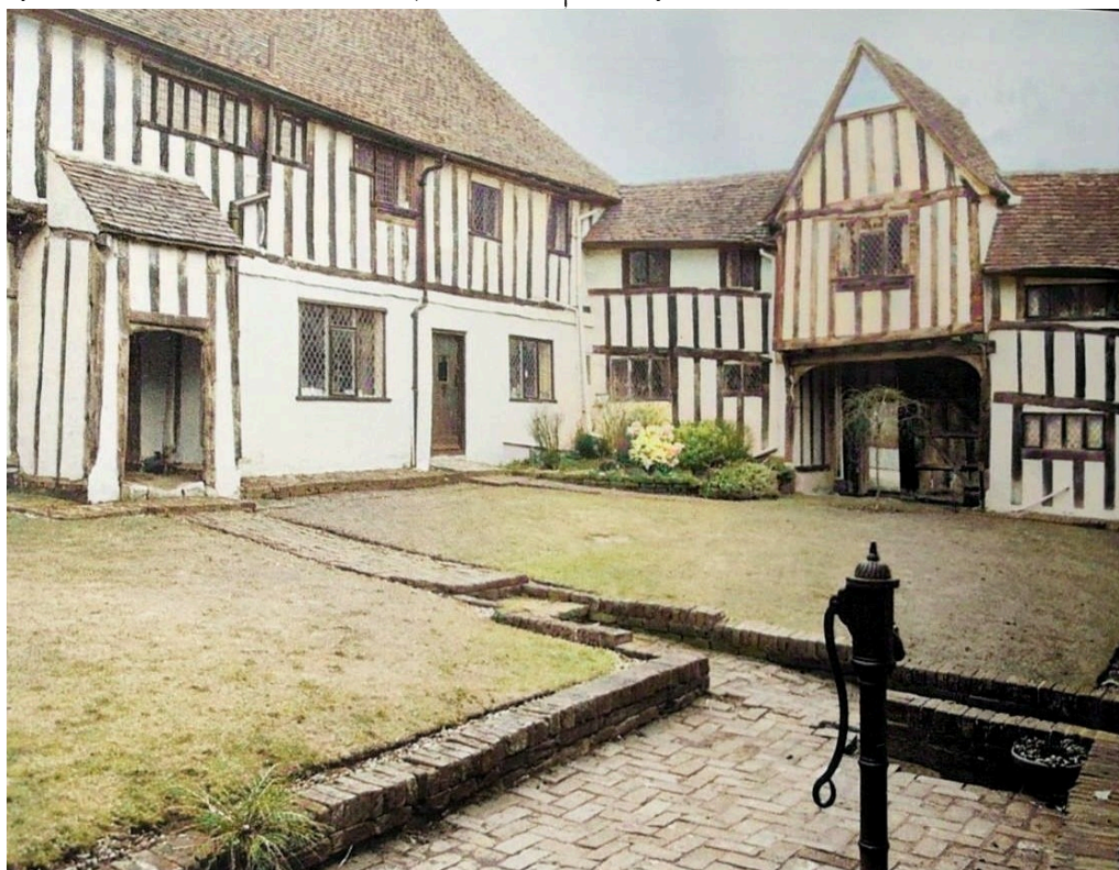
Courtyard after restoration.
